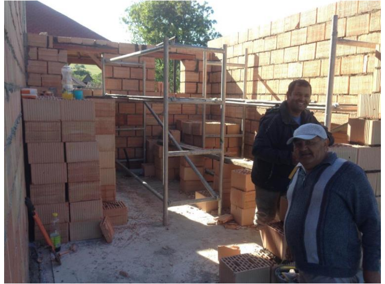
Building work in progress
