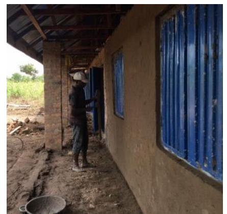
Plastering, windows and flooring
