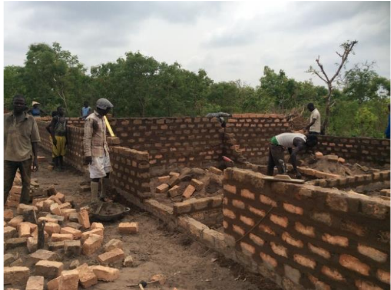
Building work begins
