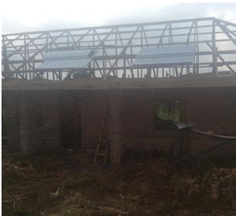
Roof timbers fixed
